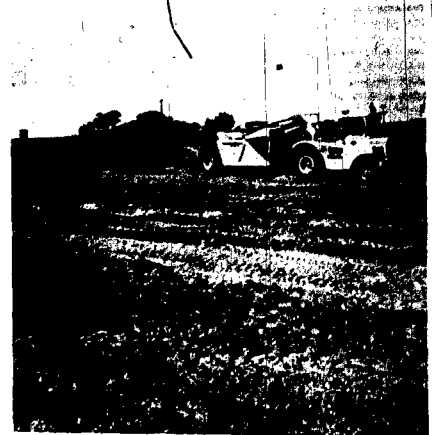
A TOURIST PARK is under construction just off Highway 33 on the west edge of the Wayne Municipal Airport and will cover a two and one-fourth acre area. The project is being sponsored by the Wayne Lions Club, according to Willis Johnson, Club president. Dirt is being hauled from the Merlound Lesman property two miles east of town by the Milo Meyer construction company. One of the heavy equipment units is shown unloading fill dirt on the park site. Johnson said Friday that plans call for seeding the area in blue grass and providing restrooms for tourists stopping to camp overnight in camping trailers.
